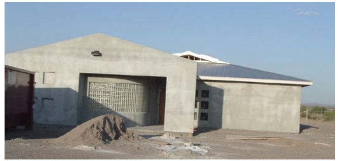
FIRRP building in progress; the Project's new home is nearly complete.
